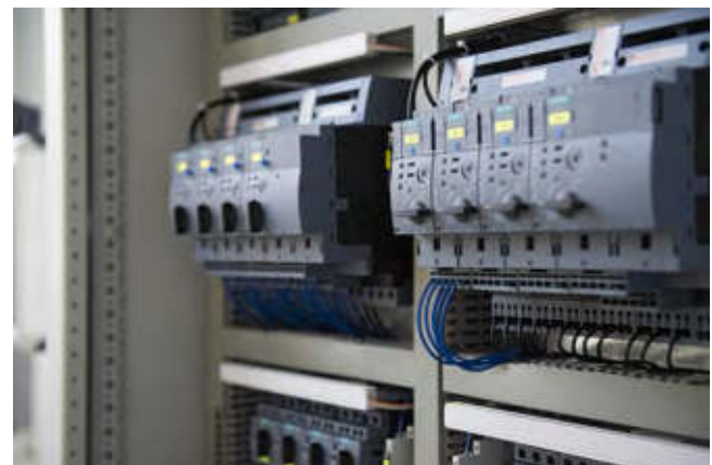
Connection of a motor starter group made up of three 3RA64 direct-on-line starters and one 3RA65 reversing starter
