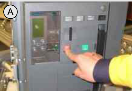
Fig. A: Press the off button on the breaker Fig. B: Key lock key rotate anti clock wise Fig. C: Device locked out
