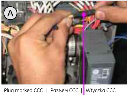
Fig. A: CCC-Plug assembly Fig. B: CCC-Coil assembly Fig. C: wiring position Fig. D: Closing Coil assembly Fig. E: Secondary disconnect plug Fig. F: Remove dummy button screw Fig. G: Extra Local ON-Pushbutton assembly
