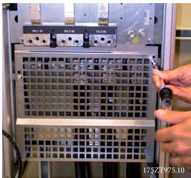
Illustration 3.21 Mounting of EMC shield.
